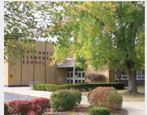
Southwest Elementary School is one of six schools and an administration building in Greenwood, Indiana that all incorporate a new comprehensive security system.
